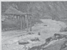
—南庄关大桥被崩塌体砸毁
